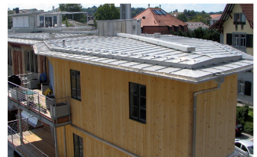
Alte Kohlenhandlung, Langenthal – Switzerland. Architects: Blum & Rossenbacher Executed using grade UGINOX Patina K41
